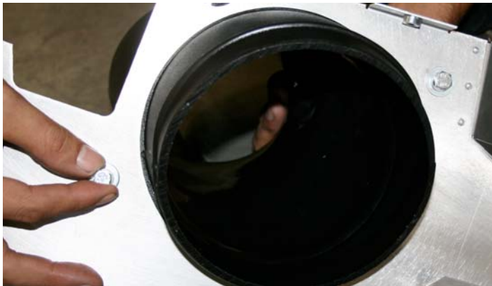
9- Install supplied hex screw, wavy washer and flat washer. Do not fully tighten.
